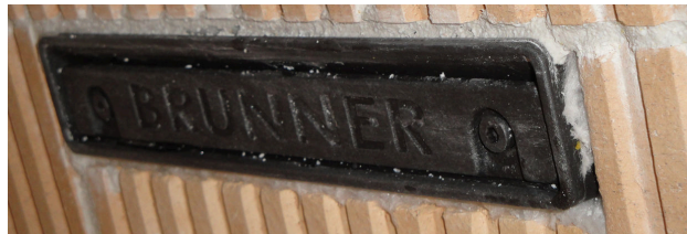
Im. 12: Combustion air nozzle with fiber felt
