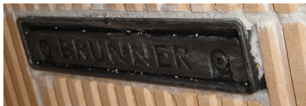
Im. 8: Combustion air nozzle with fiber felt
