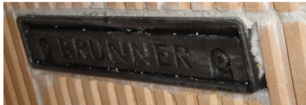
Im. 12: Combustion air nozzle with fiber felt
