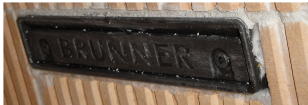
Im. 8: Combustion air nozzle with fiber felt
